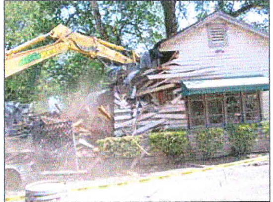
Demolition of Frank Family's old Tasting Room — the End of an Era
